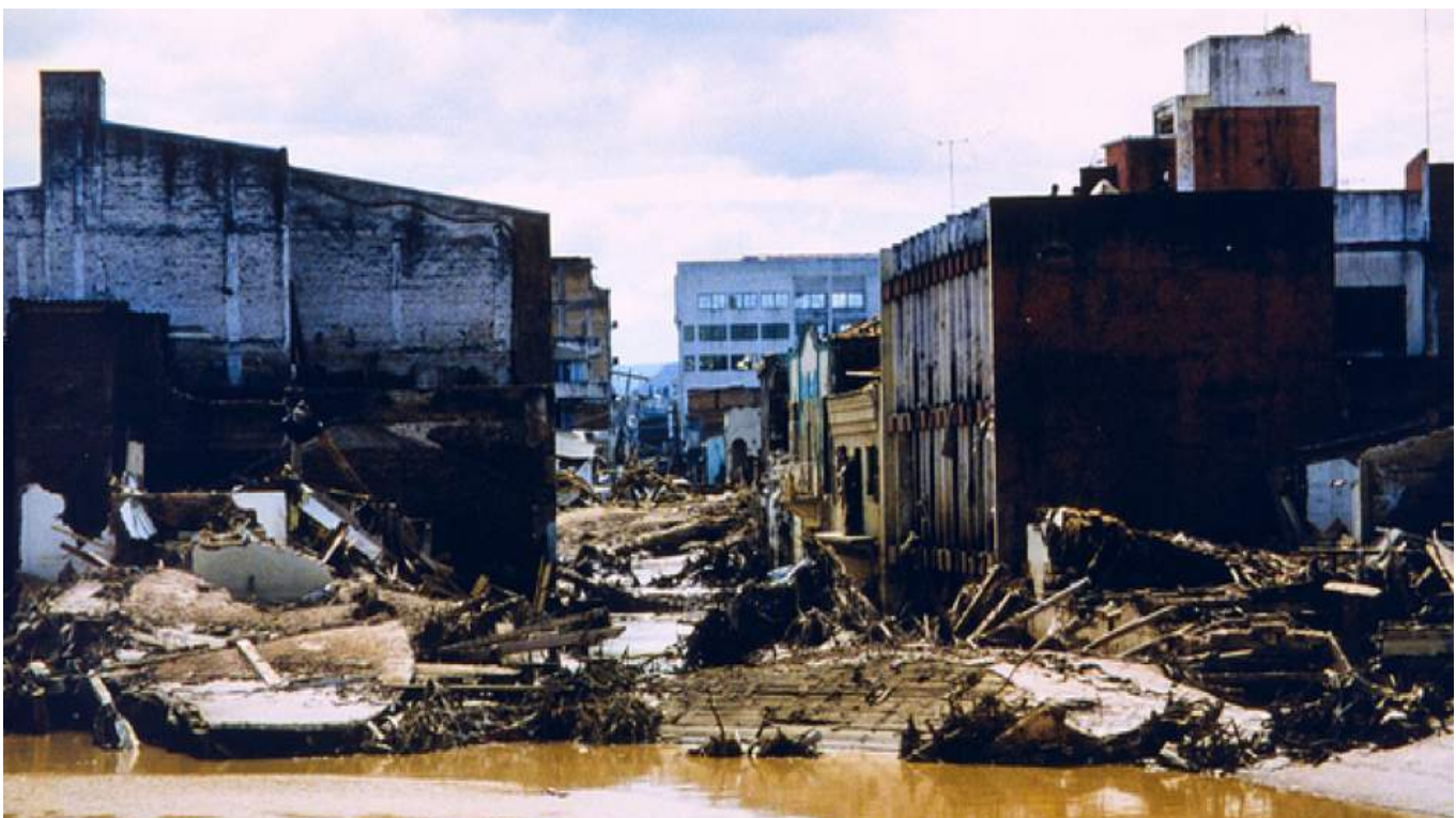
Flooding on the Choluteca River following Hurricane Mitch / NOAA Photo Library / Flickr / Creative Commons
